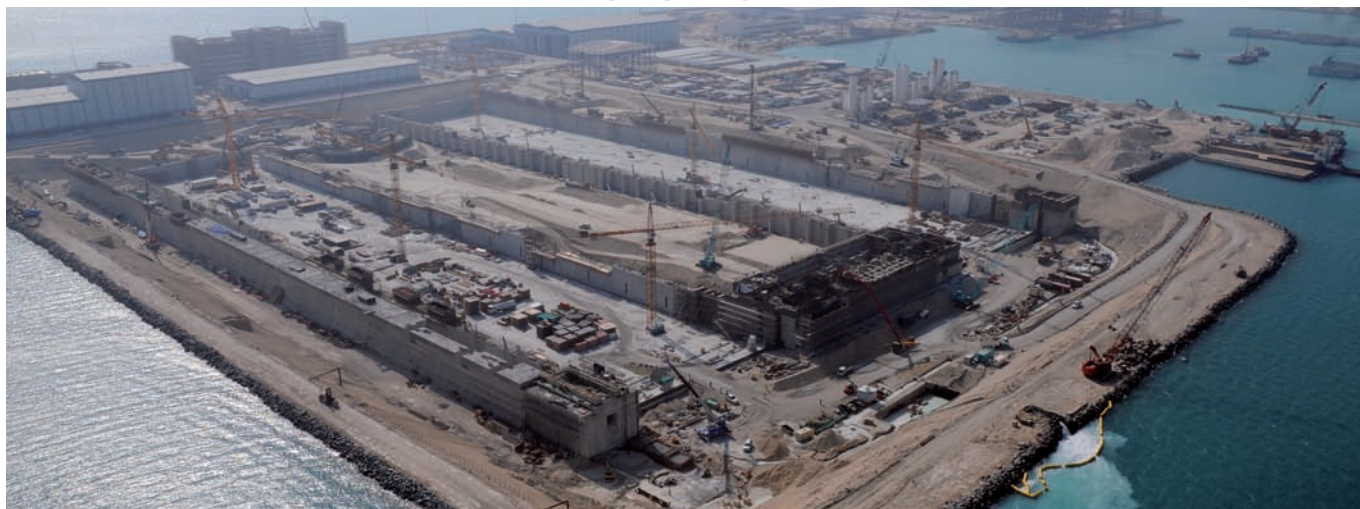
Nakilat Ship Repair Yard Phase 1, Dry Docks Under Construction
